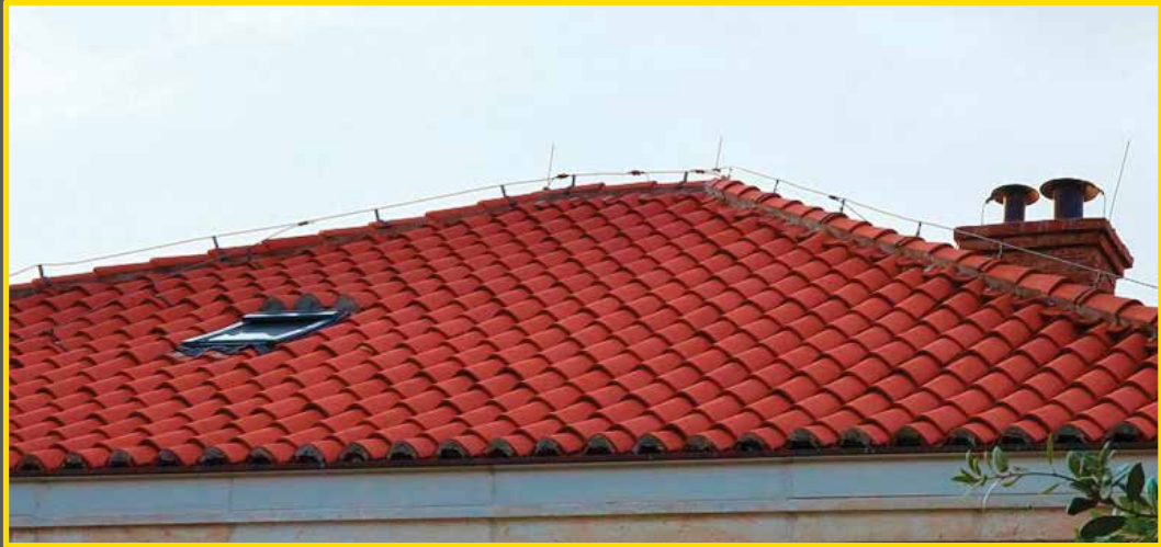
FIGURE 6: Lightning installation
