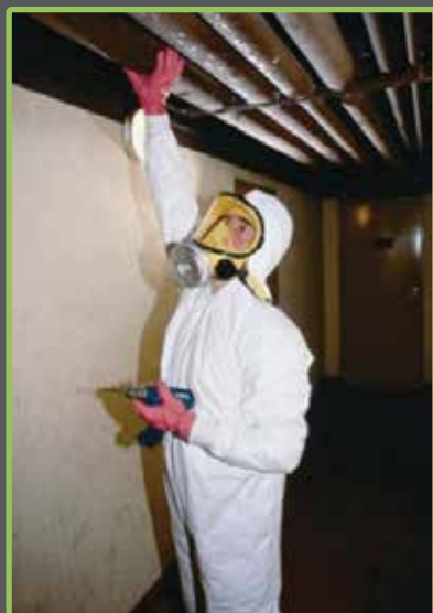
FIGURE 24: Necessary and mandatory equipment for work with asbestos
