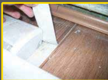
FIGURE 13: Damage of the PVC floors and baseboards
