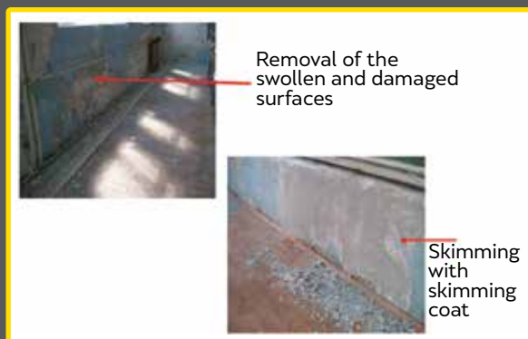
FIGURE 9: Wet spots on ceilings and walls and their removal
