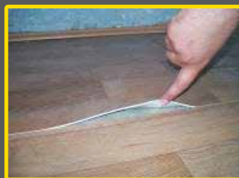
FIGURE 13: Damage of the PVC floors and baseboards
