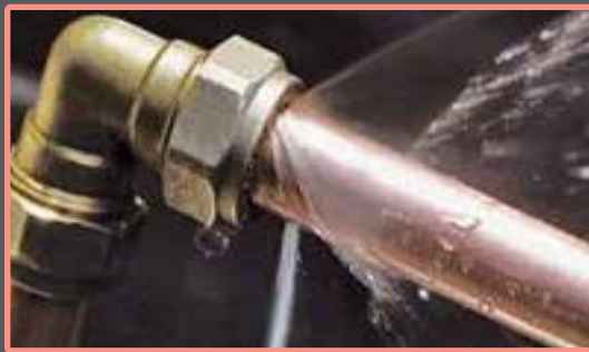
FIGURE 21: Leakage in joints and radiators
