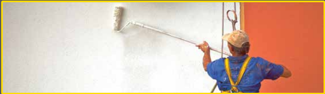
FIGURE 10: Painting internal walls with final layer of paint
